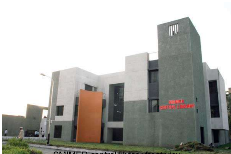
SMIMER central library front view (/smimer/Images/Facilities/central-library-1.jpg)
