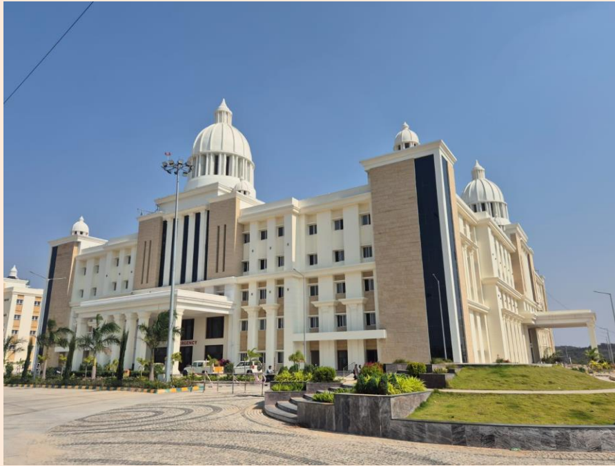
Hospital block at Arroru campus
